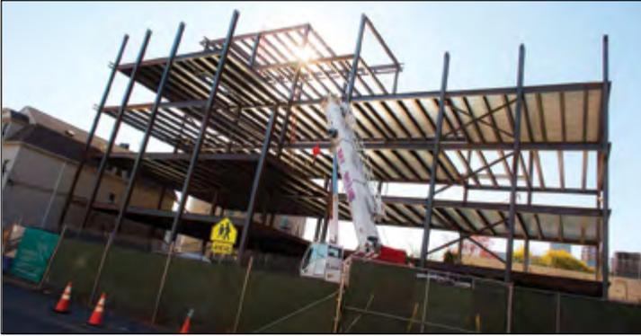
Installation of steel beams on the STEM Building taking place in early November.
